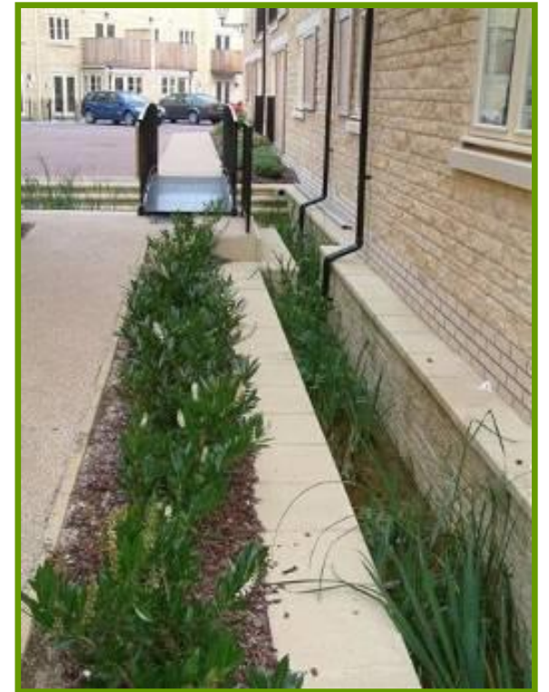
SuDS scheme at Stamford Robert Bray Associates
